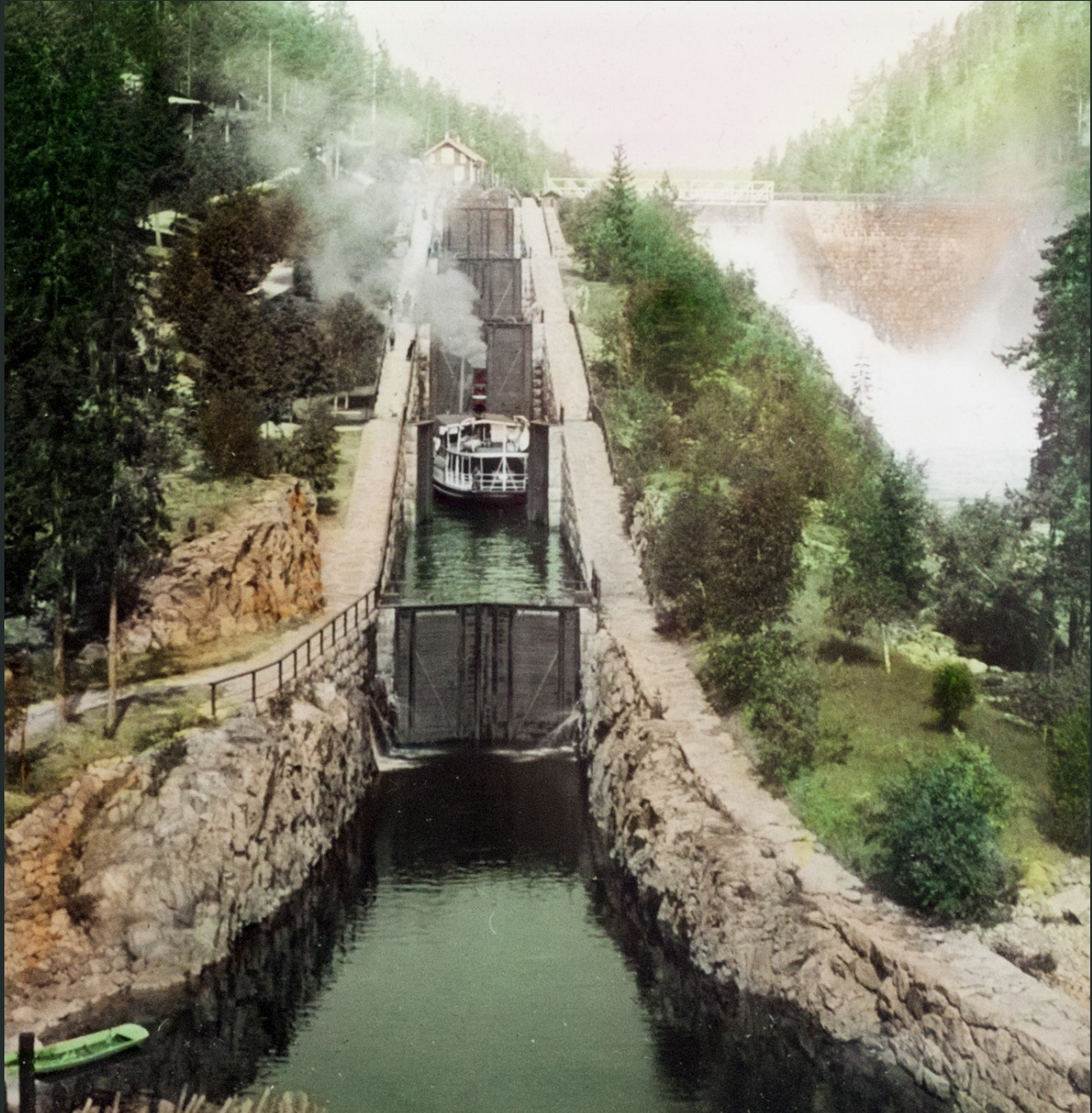
Steam boat climbing a hill, Bandak Nordsjo Canal
